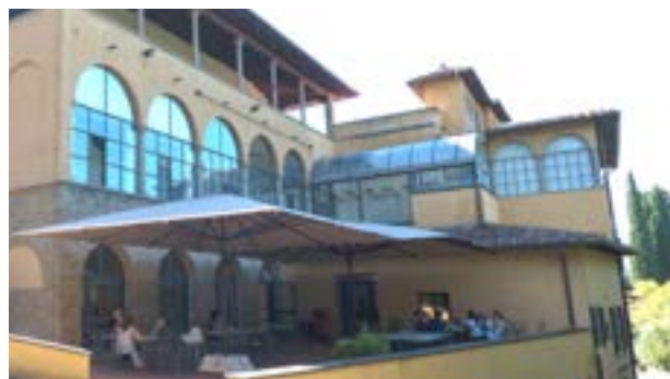
View on the terrace build after the reconstruction works
