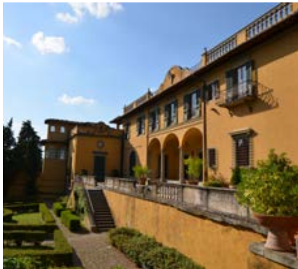
Villa Schifanoia: the main building as we see it today
